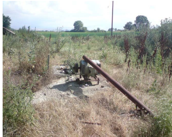
Destroyed by the CO 2 irrigating well
