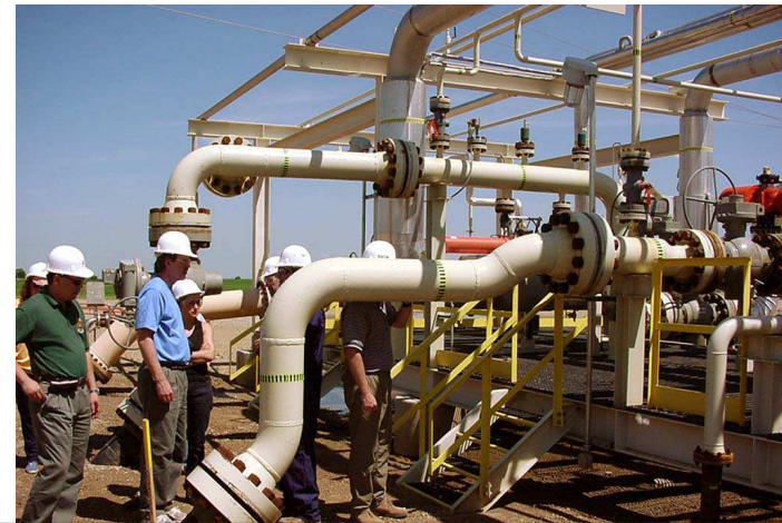
Main CO 2 pipeline enters Weyburn
